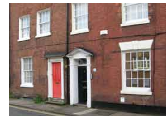
Drop in service at 10 Sansome Place
