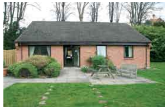
The Thorn Lodge bungalow at Osborne Court
